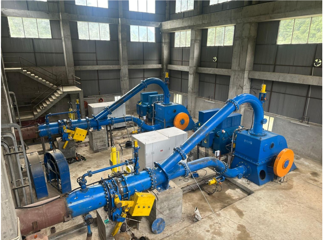
Figure 6: Completion of all erection activities of EM equipment inside powerhouse.
